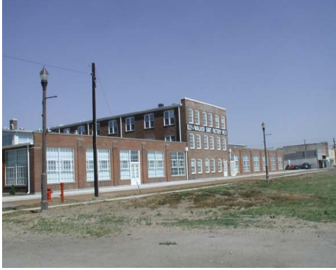
A Former shirt factory adapted for affordable housing in Downtown Kennett, Missouri.
