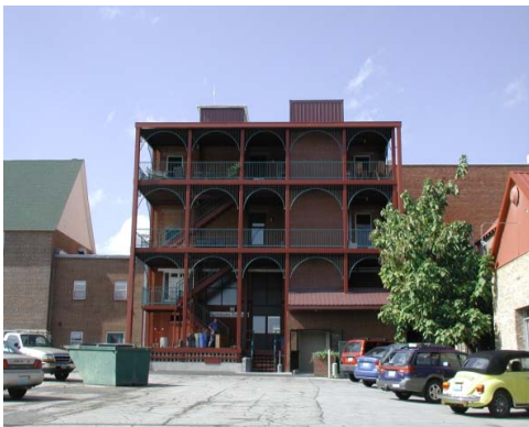
Rear view of a rehabilitated commercial building in Downtown West Plains, Missouri.
